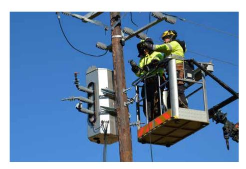
The monitoring and control cabinet that is sold with the Auguste solution is used to remotely or locally monitor and control the Auguste switch, according to the customer's requirements.
