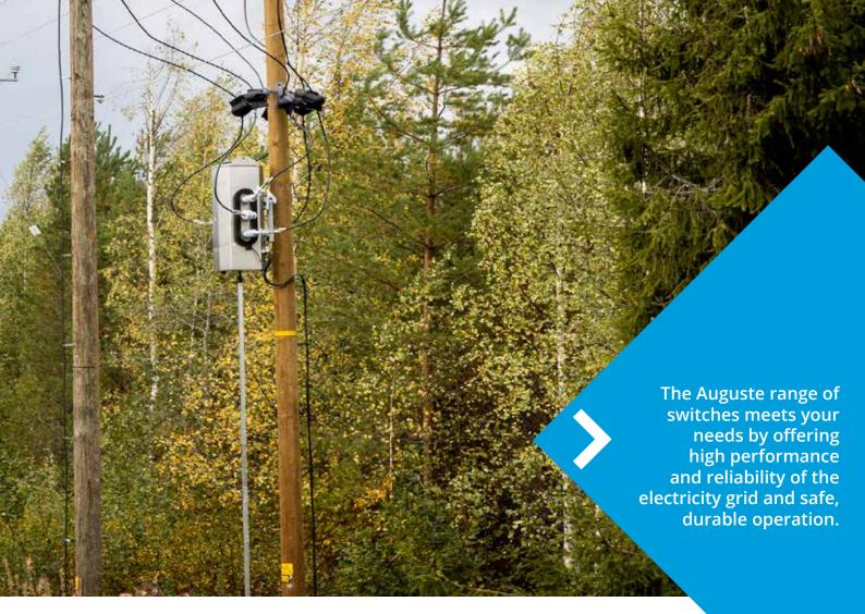
The operator can secure the grid by padlocking the switch in the different positions (open, closed or motor-operated). In addition, the new cybersecurity options of the monitoring and control cabinet protect the grid data.
