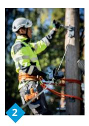
Attach the top end of the wire on the pole with a bolt. Make sure to avoid the insulator from hitting the pole.
