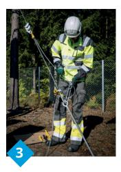
Attach the come-a-long clamp on the wire and tension it to the desired tightness with a hoist. Install the stay wire clamp on to the eye-link.
