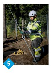
Remove the load from the hoist on to the wire and remove the hoist and the come-a-long clamp. Tighten the stay wire with adjustment nuts to desired value.
