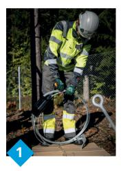
Open the kit and remove the securing tapes from the reel. Make sure to avoid the insulator from hitting the ground.
