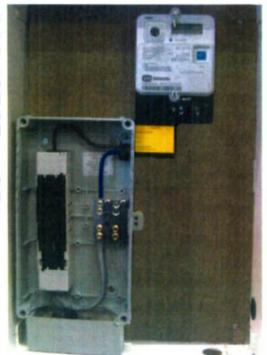
13. After the cut-out and meter have been safely energised, seal all four cover screws.
